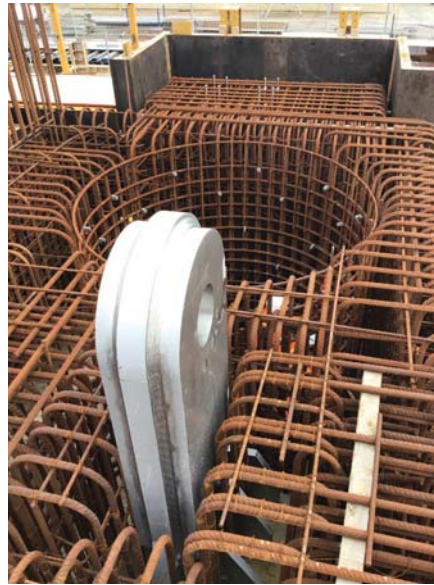
ABOVE: The reinforcement placed around the lifting lug and pile sleeve.
