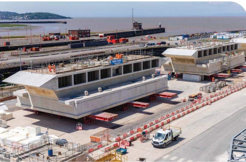
LEFT: Two of the intake heads nearing completion at Avonmouth Port.
